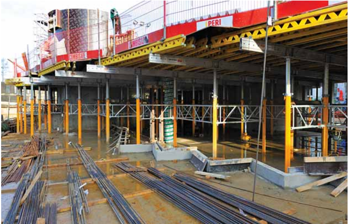
... and now coming out of the ground
