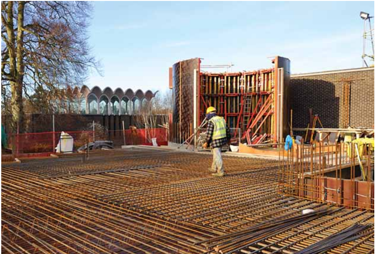
Reinforcement for the first floor
