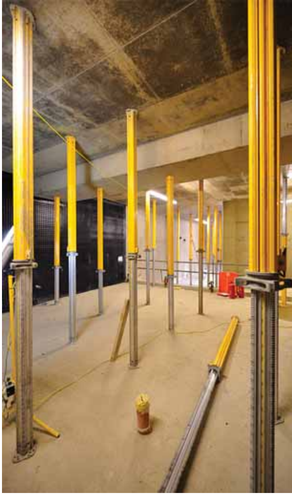
Supporting structures, in the basement...
