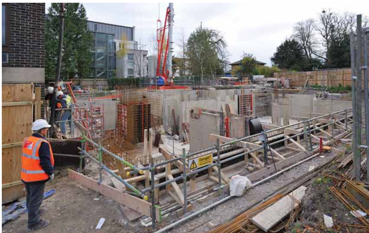
The underground structure...
